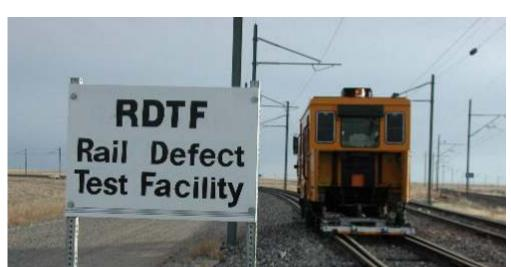
section contains a variety (over 100) of all flaw types both service and artificially induced. The track gage is between 56 and 57.5 inches (142.2 and 146.1 centimeters). Track classification is Class 3 with allowable speeds up to 40 mph (64 km/h).
